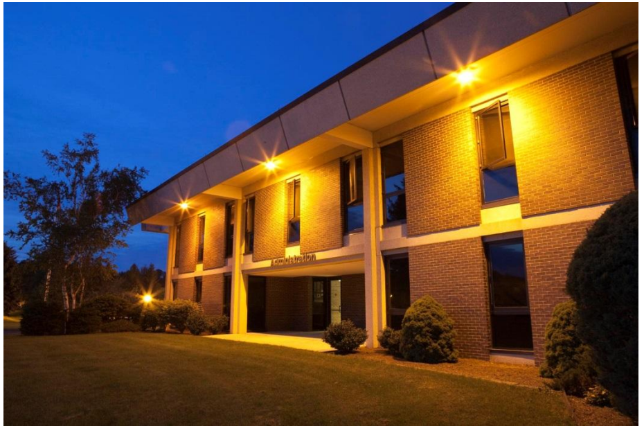
Parsons Administration Building
